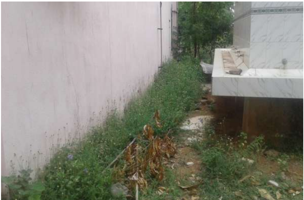
Botany Lab backside before cleaning
