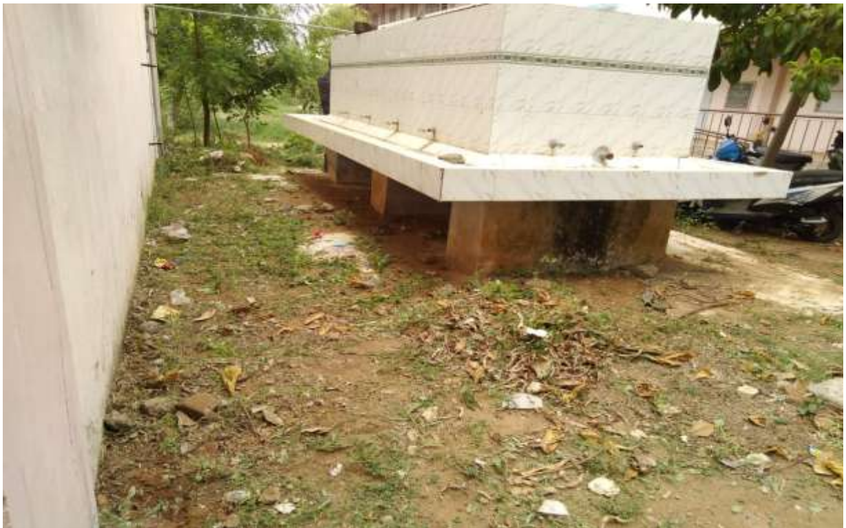
Botany Lab backside after cleaning
